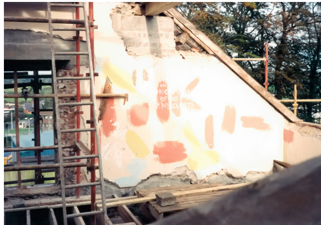
Renovating Cranagh Dhu
