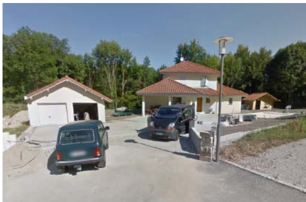
New Lebon house under construction.
