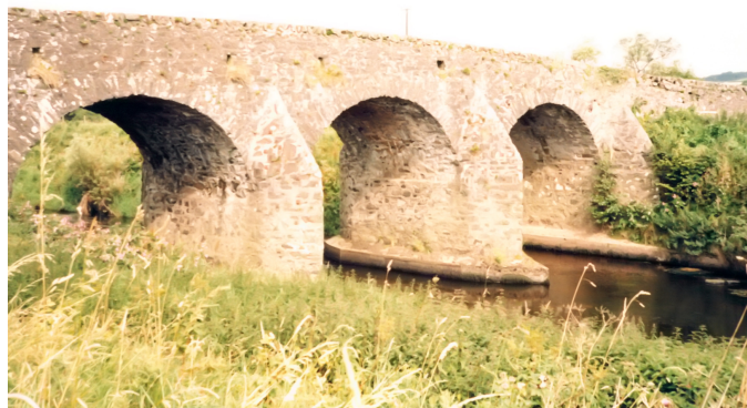
Bridge over the Moyola, Curran
