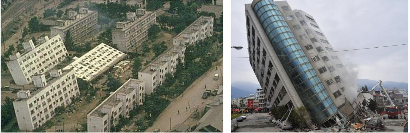
Figure 1: Soil liquefaction: Left: Magnitude 7.5 earthquake, June 1964, Niigata, Japan (Photo: Joseph Penzien.) Right: Magnitude 6.0 earthquake, February 2018, Hualien, Taiwan (Photo: CNA).
